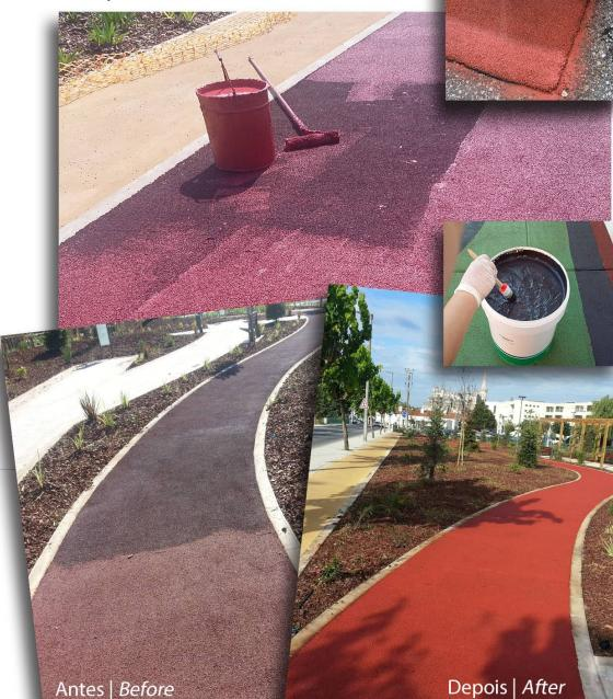
EcoRecover is a rubberized flooring recovery system, such as playground floors (plating or "in-situ"), cycle lanes and eco-run tracks in elastic materials. There are some problems associated with the playground floor, such as:
